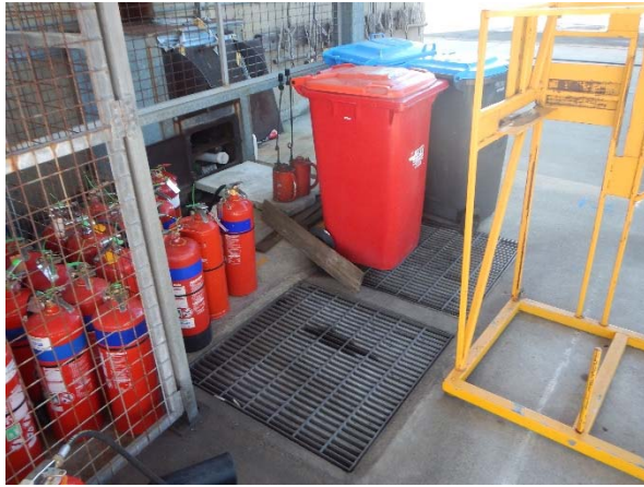
▲ Photograph 1: A drain and fire extinguishers holding cage located at the former truck wash behind the training tower on the western boundary.
