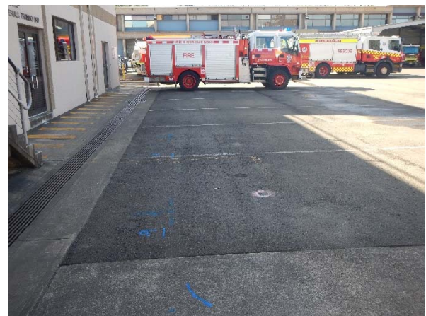
▲ Photograph 16: The drain running alongside the training centre with a groundwater monitoring (BH9A) well in the foreground installed by Douglas Partners.
