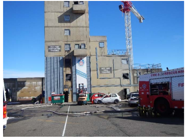
▲ Photograph 14: The training tower located adjacent to the fire training area where foam was used in the basement of the building.
