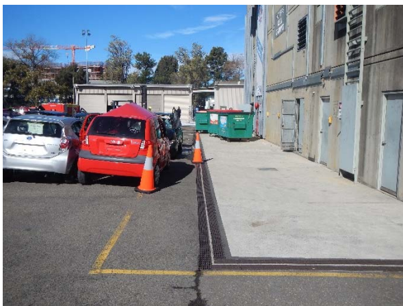
▲ Photograph 15: The drain running adjacent to the training tower. Cars that are used in training exercises nest to the training tower
