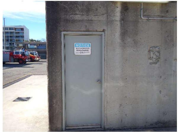
▲ Photograph 20: Storage area that may have stored AFFF within the training tower.
