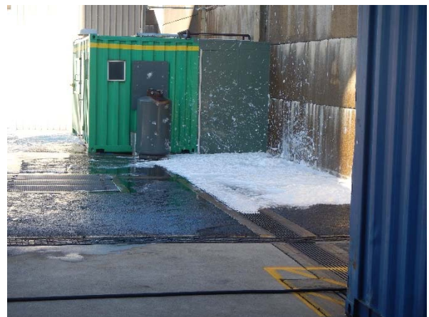
▲ Photograph 18: Training foam draining into the drain in the fire training ground.
